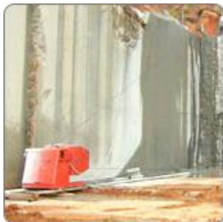
1. Granite Quarry Cutting
